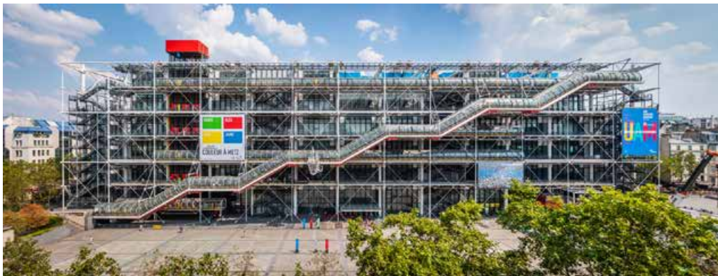
Imagen 16. Piano&Rogers Centro Pompidou Fuente: Harrouk, Christele. Pompidou Center to Close Completely for Renovations during 3 years 2021. ArchDaily
